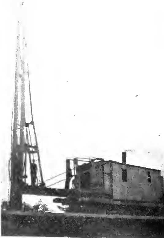
Pile driver in position for driving.
